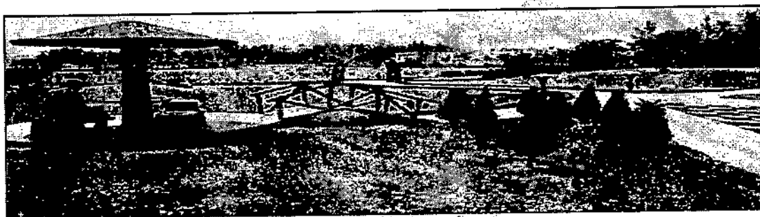
Figure 6: Dry Ash Mound at NCTPS, Dadri (After Stabilization and Plantation)
