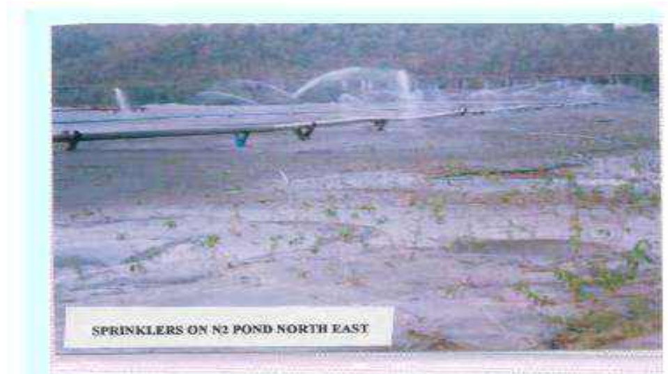
a) Safe Disposal for Control of Fugitive Dust with Sprinkler
